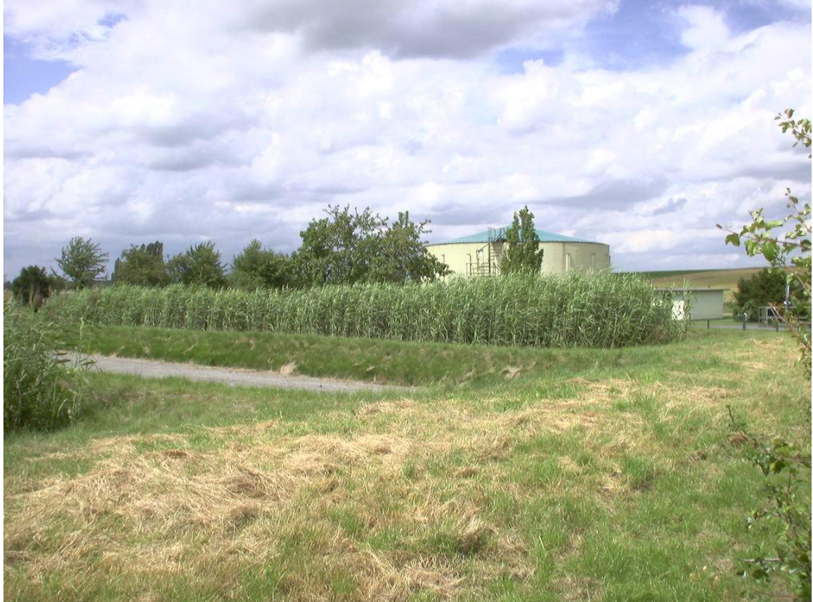
Gadenstedt, reed bed 1, with trickling filter plant in the background
