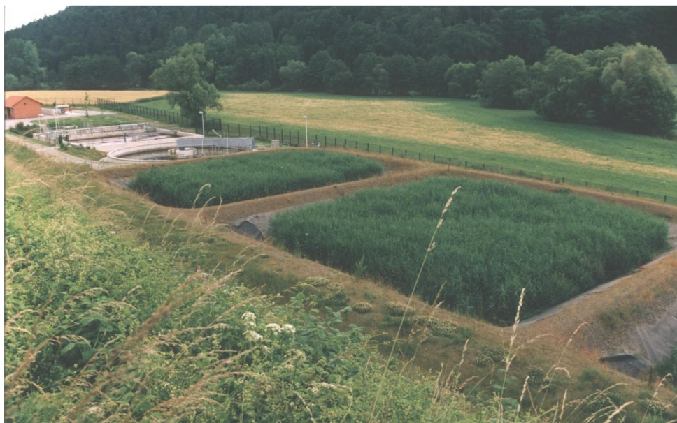
Reed bed dewatering Naumburg, beds 1 and 2, activated sludge treatment plant in the background
