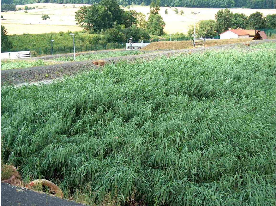
One of four reed beds at sewage treatment plant Bad Emstal (6,000 m 2 in total)
