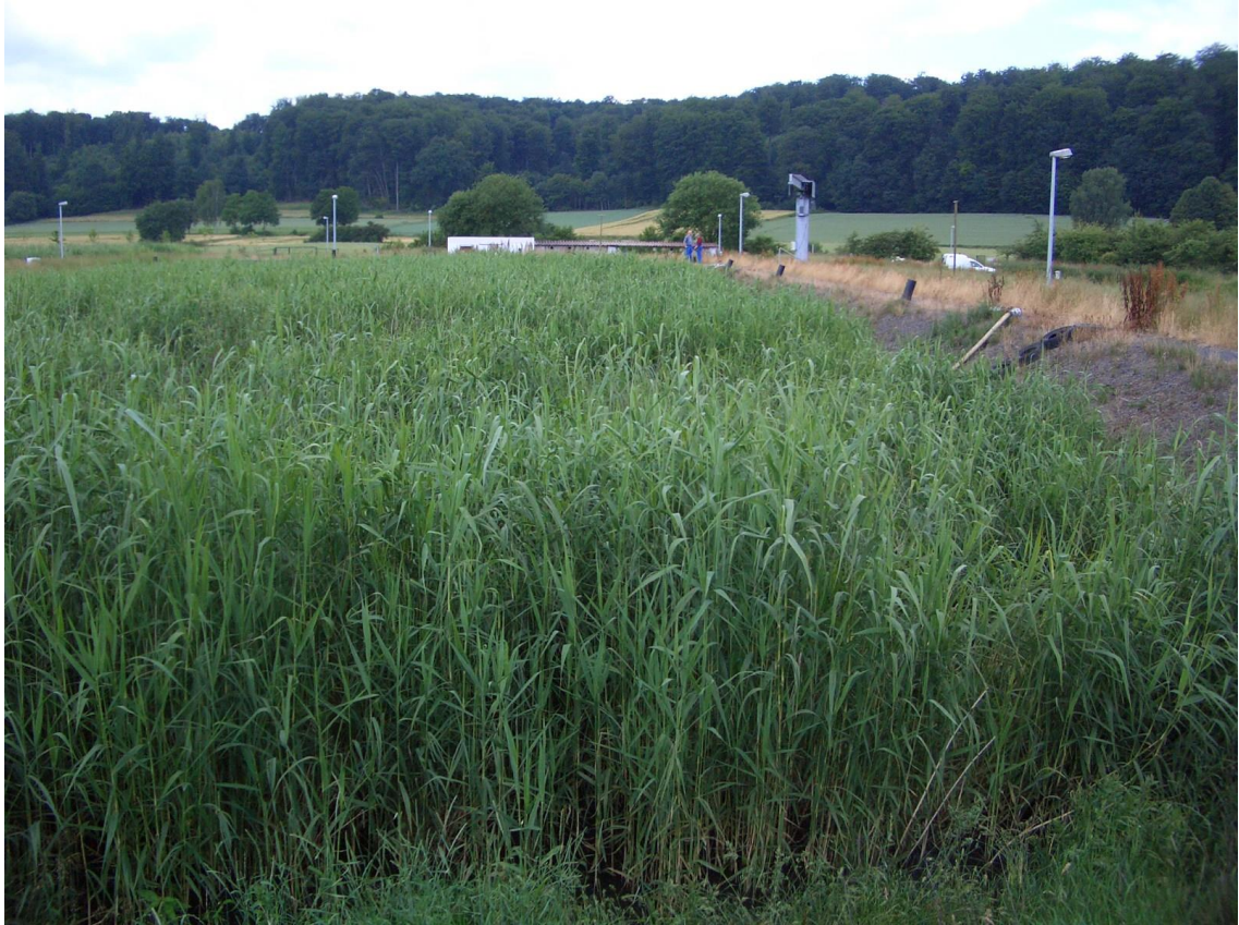
Sludge drying reed beds Fronhausen (2.000 m 2 )
