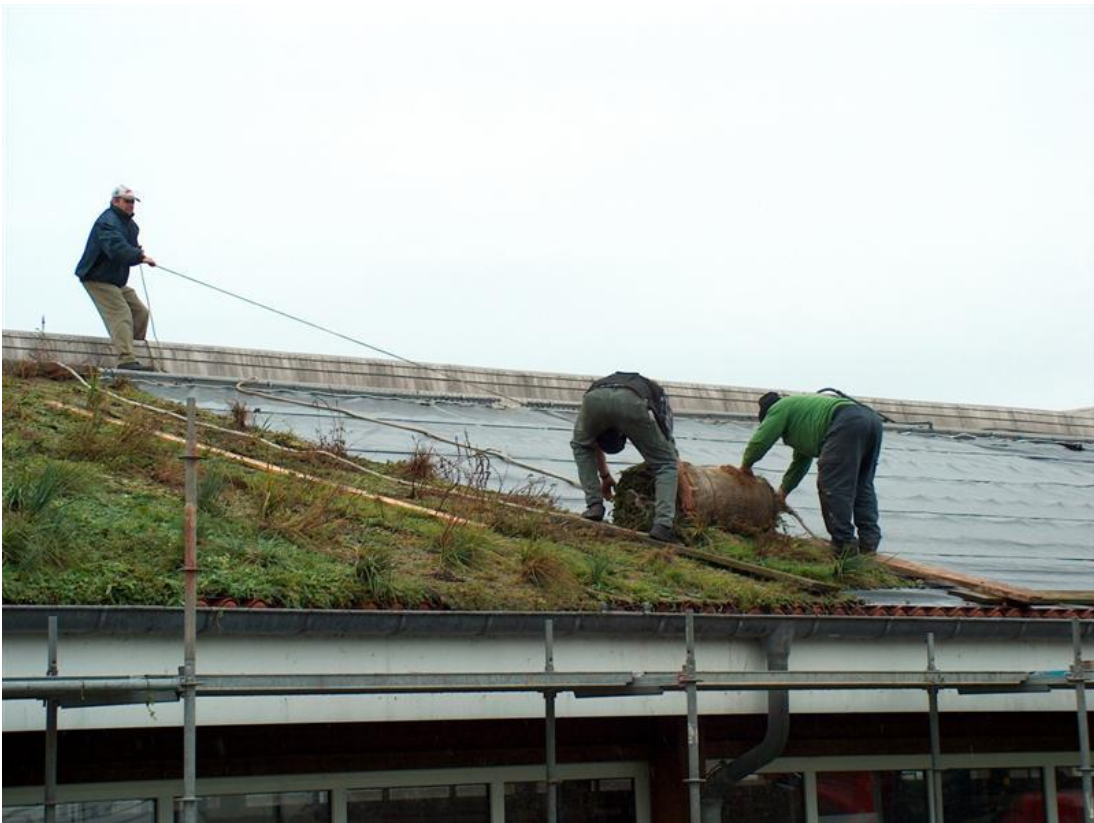
Installation of the plant carrier and water storage mats on a wetland roof.
