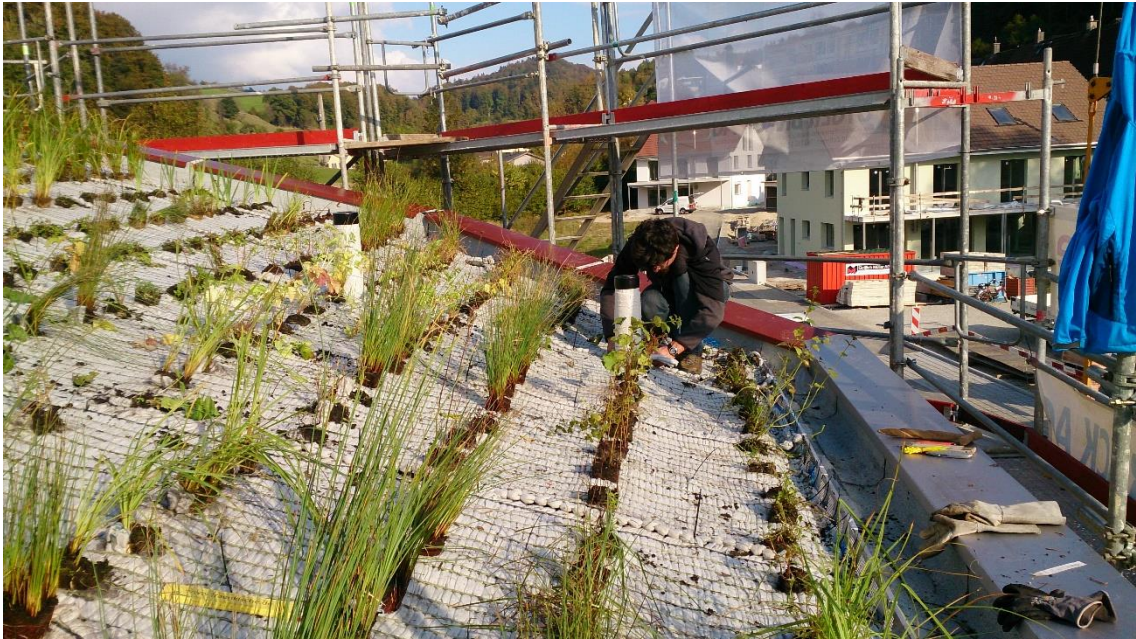
Installation of plants on a wetland roof in Zofingen, Switzerland.
