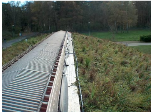
Irrigation along the ridge of the roof
