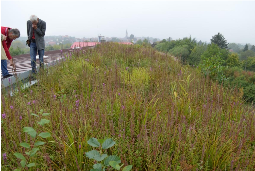
A wetland roof on a two-story office building in Jena, Germany.
