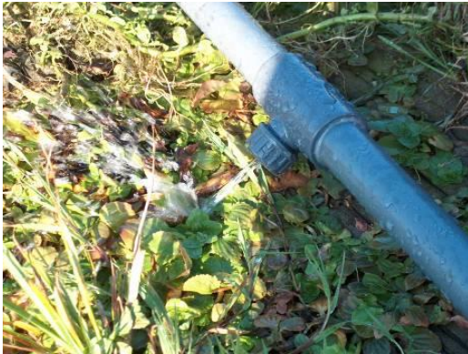
Outlet drippers of the water feed system
