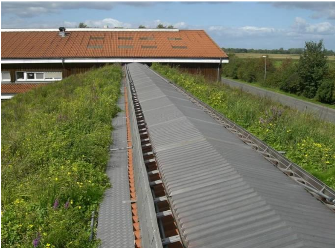
A cowshed roof covered with helophyte (marsh plants) mats in Brunswick, Germany (2006), designed by Blumberg Engineers and constructed by Rhizotech (900 m 2 ).
