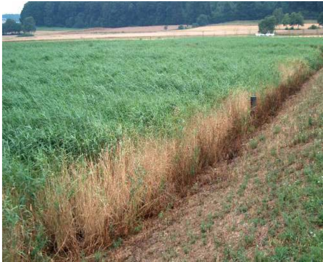
Constructed wetland in Germany
