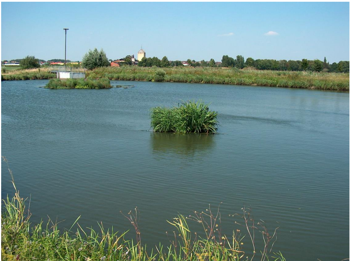
Stormwater treatment biotope Gadenstedt, Germany
