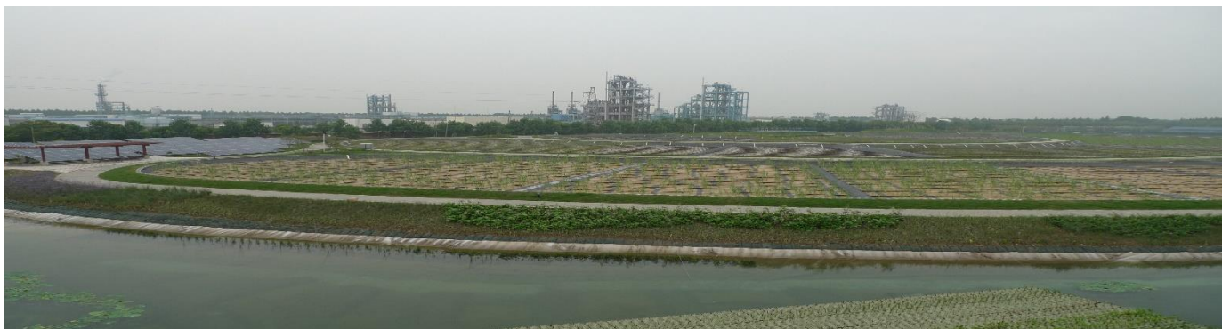
Vertical subsurface flow constructed wetland
